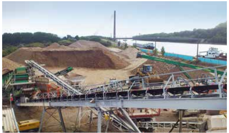
ECO-FRIENDLY CONCRETE Lanaye locks, Belgium
